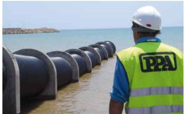
Installation of an outfall pipeline in Spain
