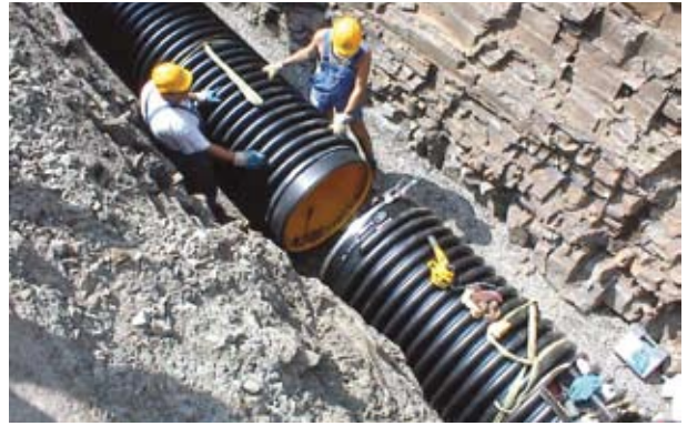
Pipe installation in Argentina
