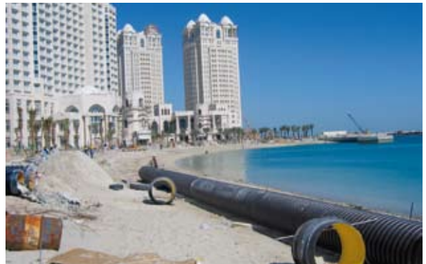
Pipe installation in Doha, Qatar
