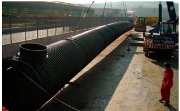
Installation of a storm water retention basin
