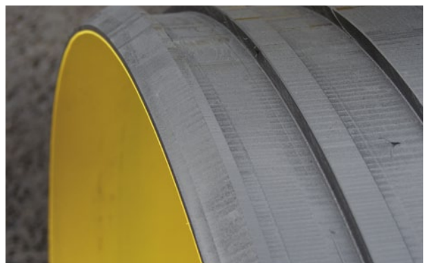
Grooves for gaskets on the pipe
