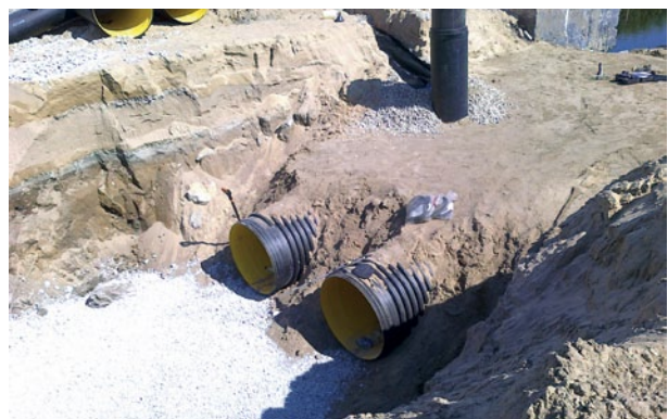
Installation of Krah pipes DN/ID1000 at a construction site
