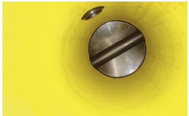
Inspection manhole for sewage DN/ID800
