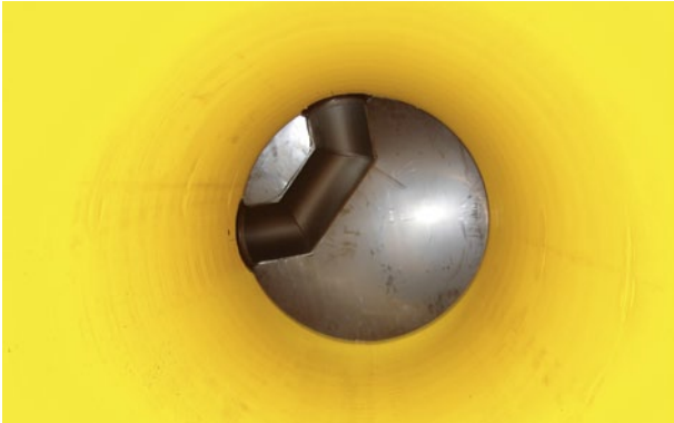
A turn inside manhole ID800
