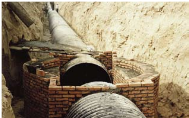
Krah pipe with a manhole - produced with bricks
