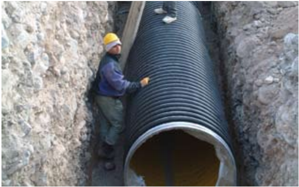
Krahe pipes installed in a very narrow trench
