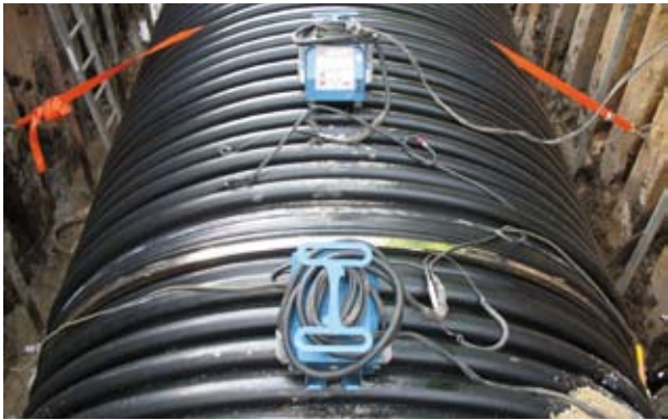
Electro fusion connection on site
