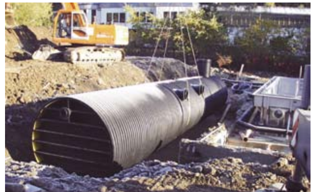
Installation of a swimming pool storage tank
