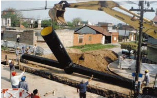
Quick manhole installation
