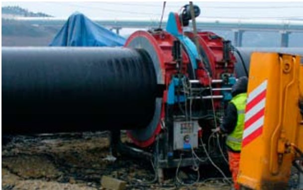
Heat element butt welding connection
