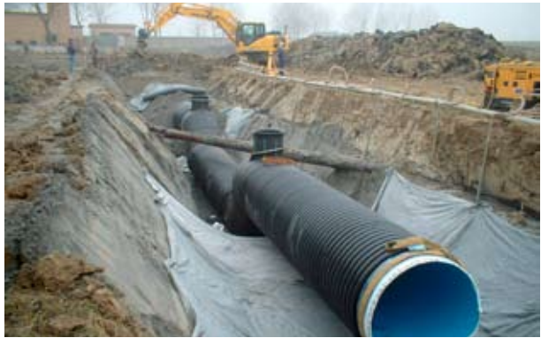
Installation of a pipe DN/ID 2000mm
