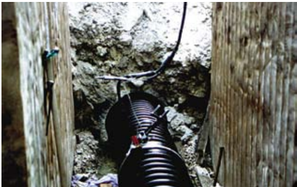
Relining of a concrete pipe
