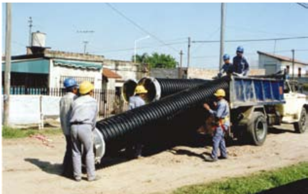
Manual unloading of a pipe DN/ID 600mm
