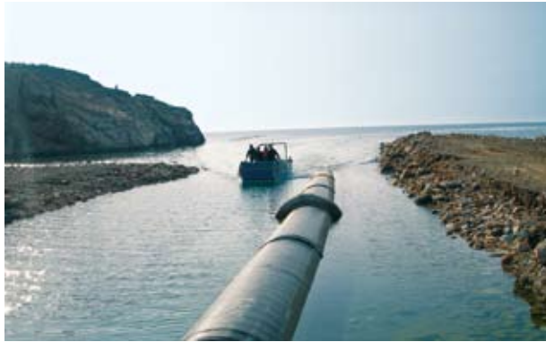
Outfall pipe line DN/ID 2000mm
