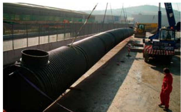
Installation of rain water tank
