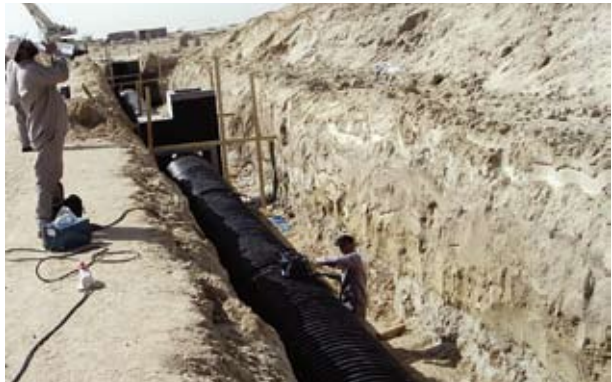
Installation of a sewage pipe with a complete manhole
