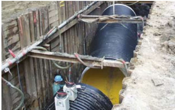
Sewer pipeline DN/ID 2000mm
