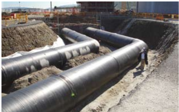
Installation of a TWIN-pipe DN/ID 2000mm with fittings
