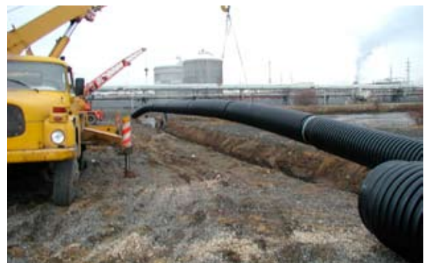
Installation of a pipe
