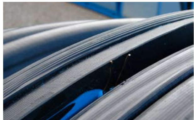
Electro fusion weld of a pipe connection
