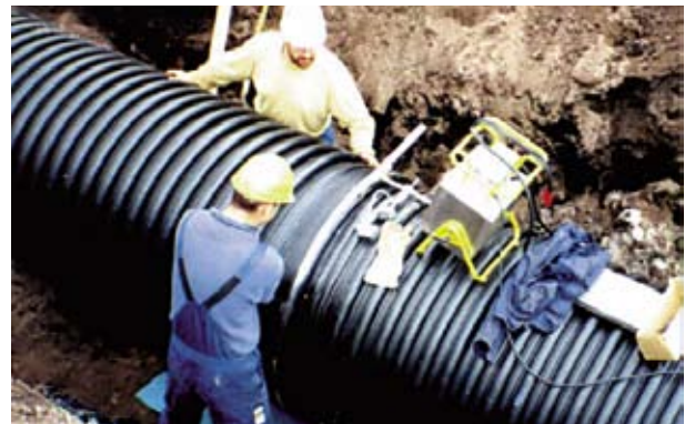
Electro fusion welding procedure
