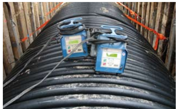
Welding of a large diameter pipe in a narrow trench
