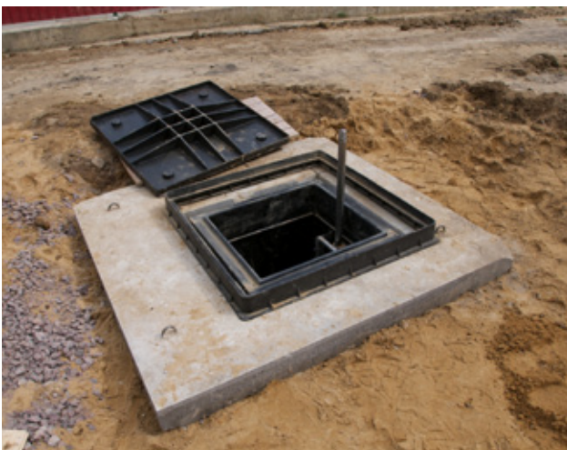
Russian Federation, Saint-Petersburg, Toksovo ID1200 H=3800 mm with a calculated body. Pumping station was installed under the traffic, with a cast iron cover for 40 t.
