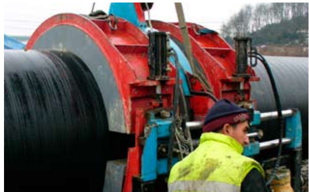
Butt-fusion of a Krah-Pipe DN/OD 1600mm SDR17
