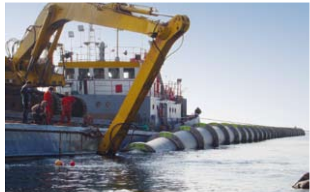
Outfall pipeline DN/ID 1800mm
