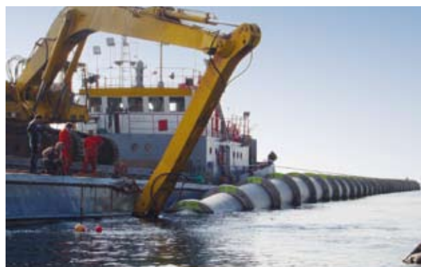
Uputatav torujuhe DN/ID 1800mm
