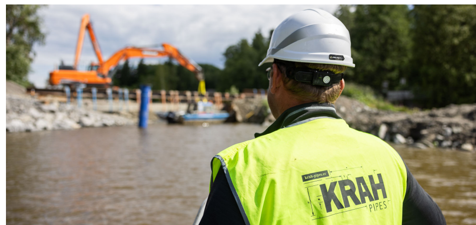
Tampere outfall project - DN 1800 pipes installed across lake, Finland (2024)
